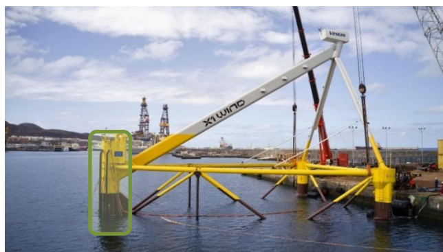
Figure 2 Boat Landing X30 Platform
