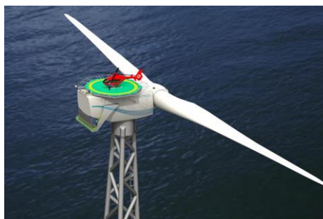
Figure 5 Helicopter Access 2 Bladed Turbine
