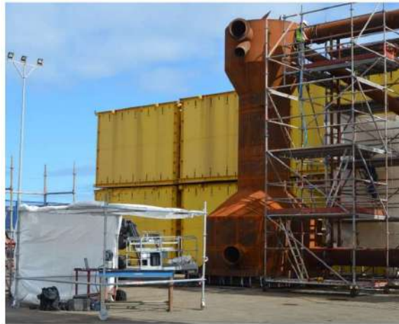
Figure 7 Main Column of Prototype during Assembly
