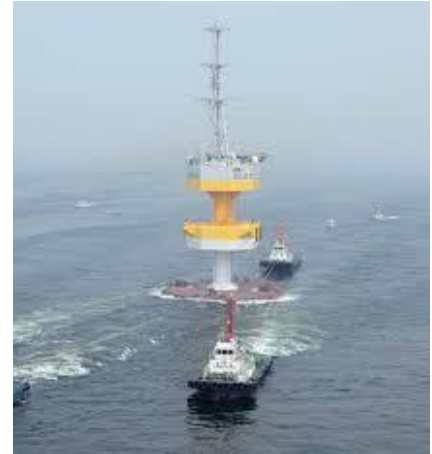
Figure 10 Advanced spar design of the Fukushima Hamkaze showing underwater section (left) and floating substation (Fukushima Kizuna) with the advanced spar design being towed to site (right). [25]
