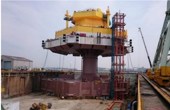
Figure 10 Advanced spar design of the Fukushima Hamkaze showing underwater section (left) and floating substation (Fukushima Kizuna) with the advanced spar design being towed to site (right). [25]
