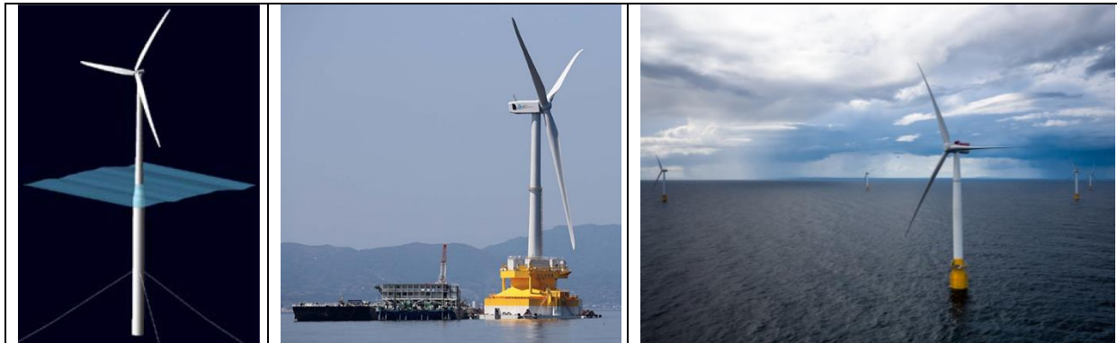
Figure 9 Spar buoy concepts: the OC3-Hywind (left) taken from [24]; 5MW downwind advanced spar (center) [25], and Hywind Scotland (right).
