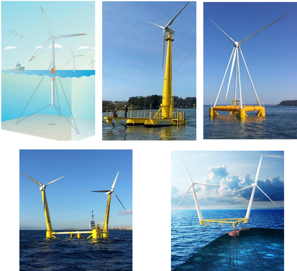
Figure 13 Examples of hybrid concepts, top row from left to right: TLB conceptual design, source: [2]; BlueSATH demonstrator; and Eolink demonstrator, source: [62]. Bottom row, from left to right: W2Power demonstrator, source: [63]; and Hexicon concept TwinWind, source: [64].
